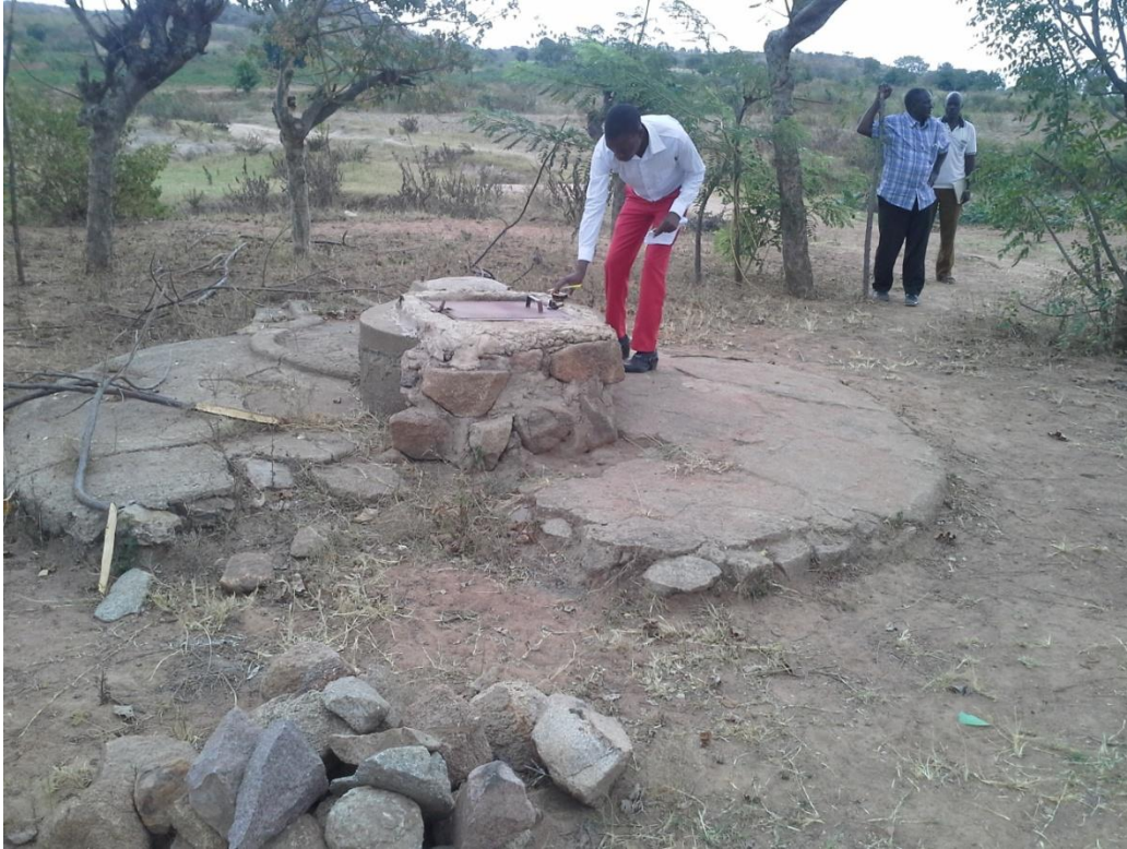
Shallow ell that was constructed on 1972, it has depth of 12Ft. = 4M. It has gone dry,
